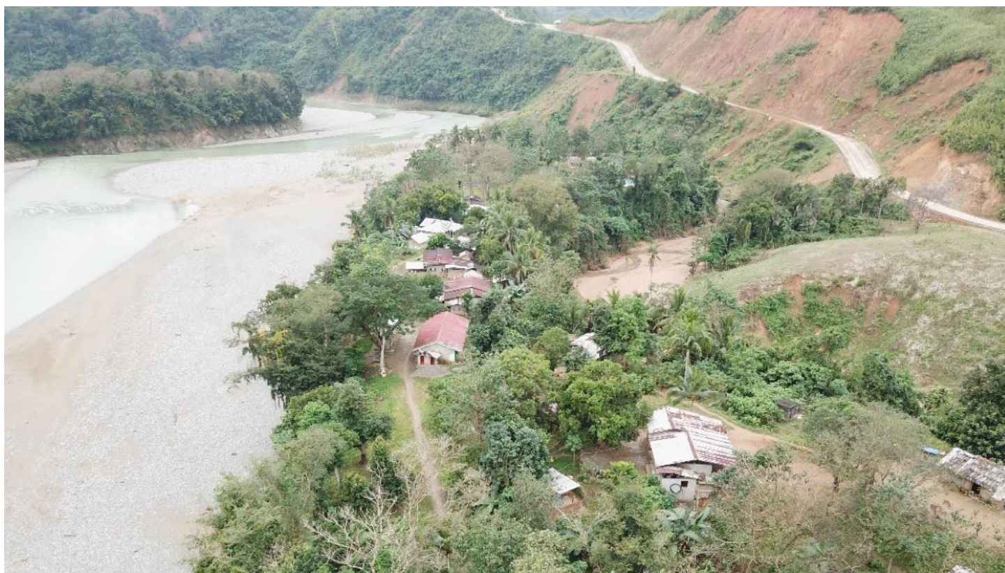
Aerial photo ti project site
